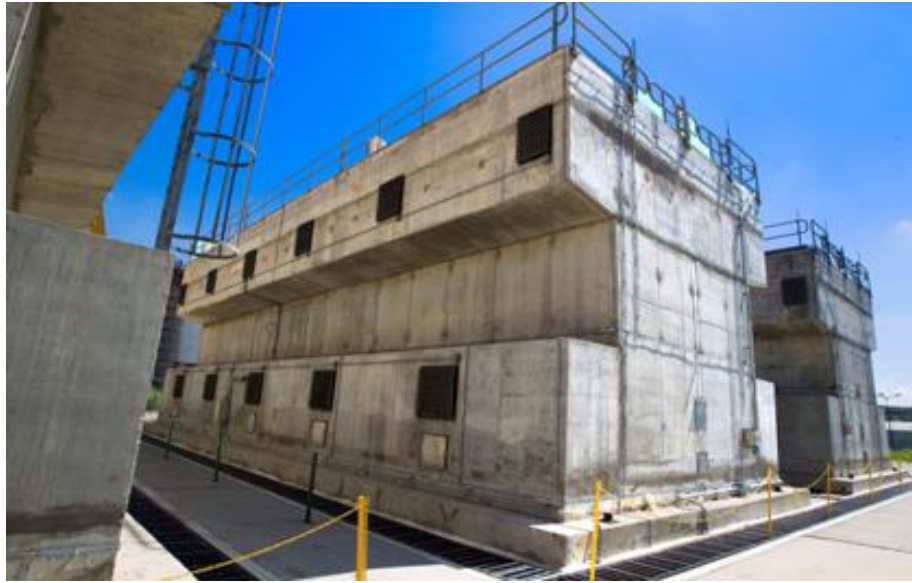
Fig. 1.4 Intermediate Dry Spent Fuel Storage
