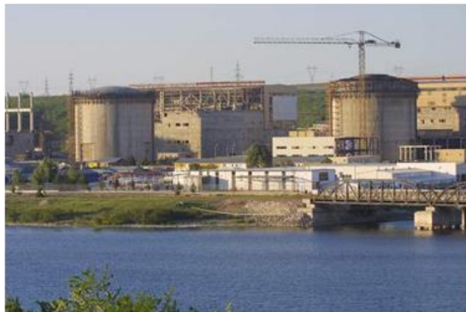
Fig. 1.2b Cernavoda NPP Units 3 and 4
