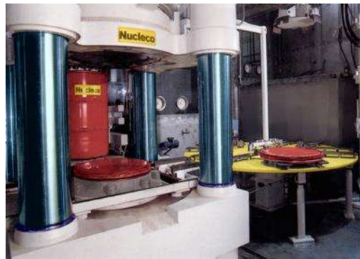
Compacted drum height measure and pellet positioning in overpack
