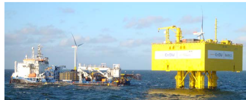
Cable Pull-in at OSS Baltic 2 (50Hertz, DE)
