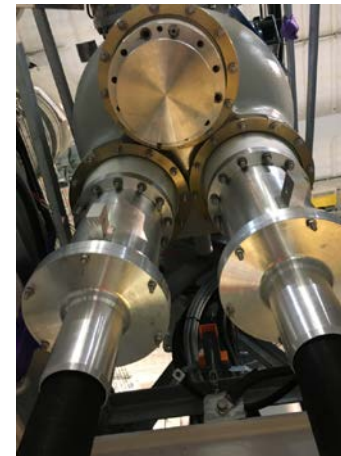
150-kV GIS Termination works, 2018
