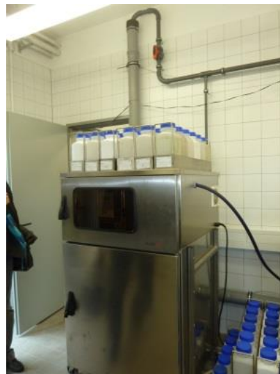
Figure 31. Automatic river water sampling system
