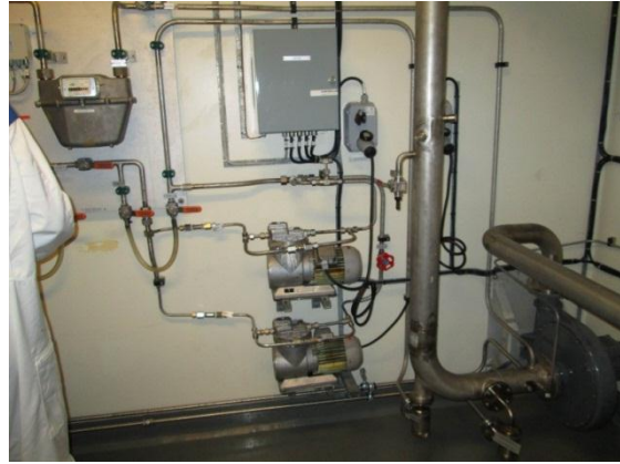
Figure 3. CLAB main stack and air discharge sampling and monitoring devices
