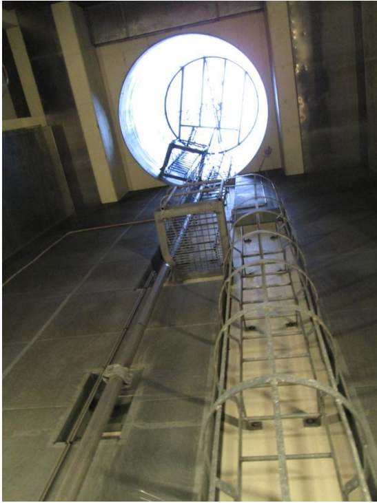
Figure 3. CLAB main stack and air discharge sampling and monitoring devices
