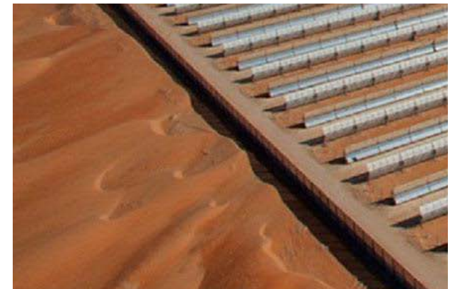
Shams 7 m high Wind Break Barriers
