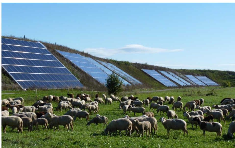
Figure 11: The 'solar wall' that forms part of the Hirtenwiesen 2 system in Crailsheim. Courtesy of: Hamburg Institute.
