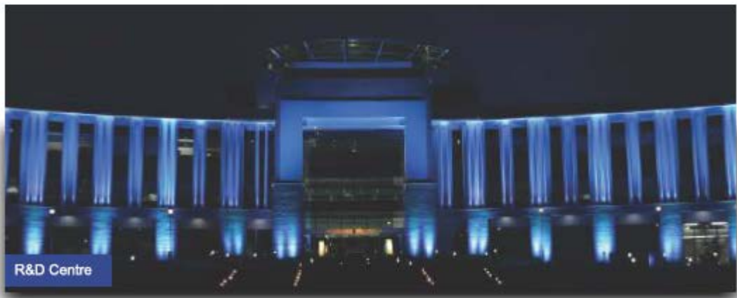
HP GREEN R&D CENTRE, BENGALURU
