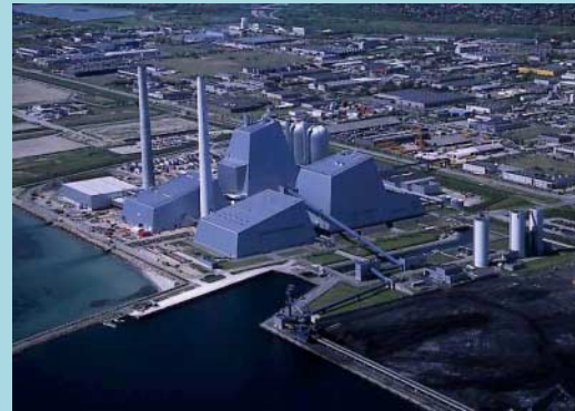
Avedøre plant in Copenhagen. Energi E2.
