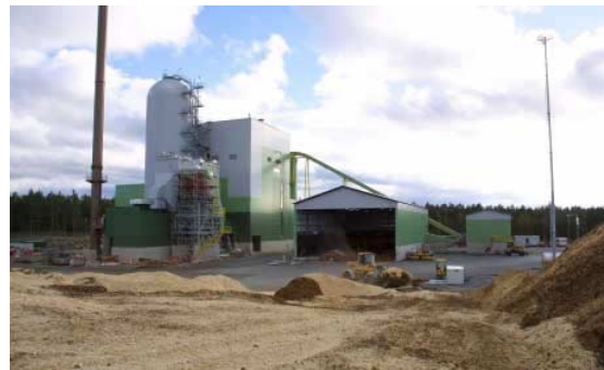
The main fuels of the Kokkola power plant in Finland are wood-derived fuels and peat, which can be stored in the fuel yard. In the basic planning, special attention was paid to a flexible selection of fuels on an extensive range of partial loading without the risk of corrosion. The Kokkola power plant is producing 20 MW e of electricity and the output of the BFB-boiler is 70 MW th . Pohjolan Voima Oy.
