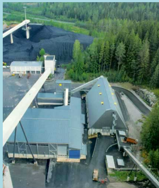
Fuel receiving stations and coal yard. Roxon.
