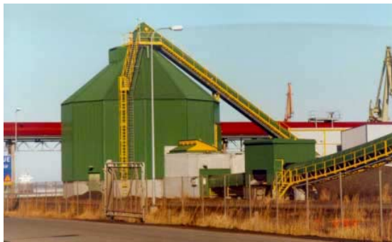
The round-bottom intermediate storage (1500 m 3 ) of a biofuel power plant. Roxon.
