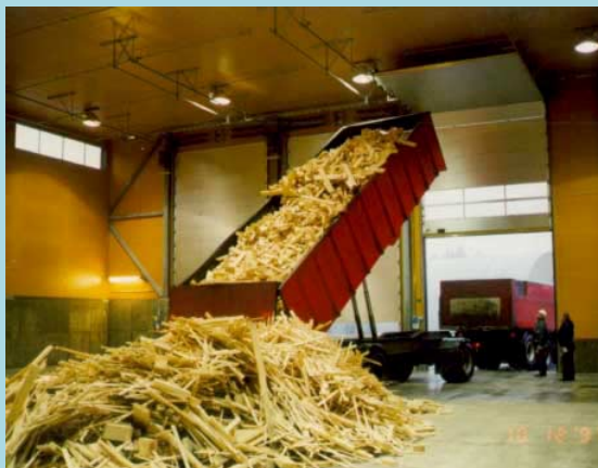
Wood fuel storage at Lahti plant. Roxon.
