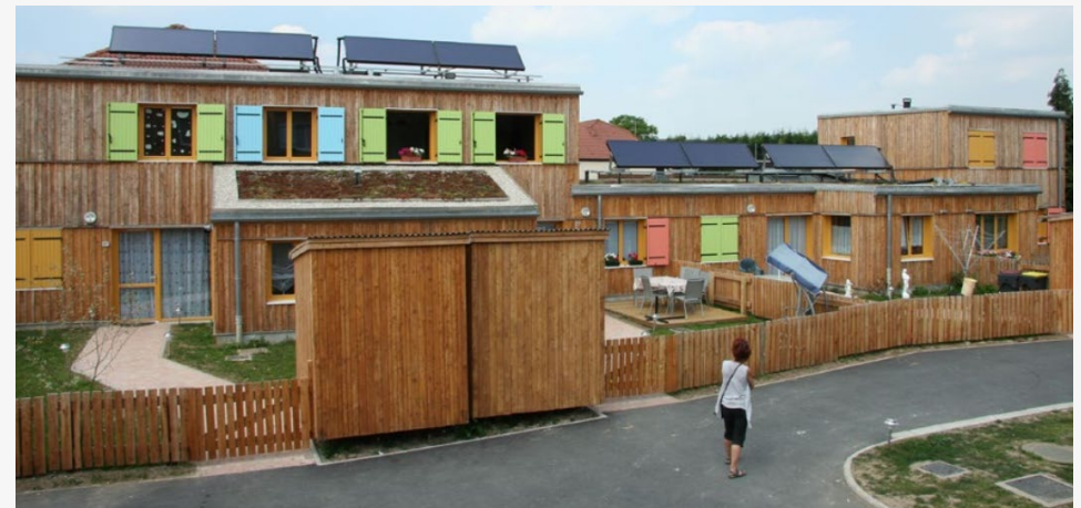
SOLAR INSTALLATIONS IN FORMER COAL MINING TOWN OF LOOS-EN-GOHELLE, DEVELOPED VIA A PUBLIC-PRIVATE-PARTNERSHIP (PPP)
