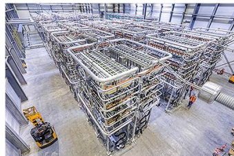
Siemens HVDC Plus for the COBRA converter stations.
