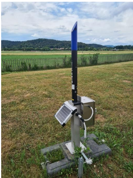
Figure 41. MIRA station at the Research Reactor
