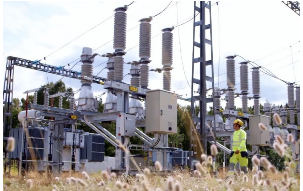
Tranås Energi, Sweden 2015 (4 units DCB LTB 72.5 kV)
