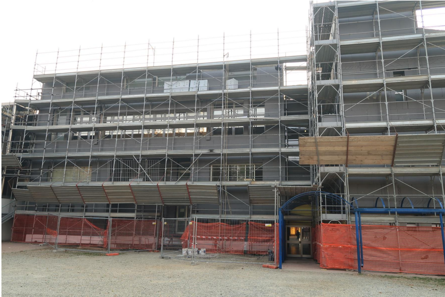
Works ongoing in the City of Volvera
