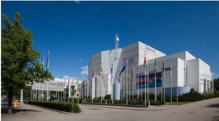
Figure 17: Total Concept pilot building- Denmark
