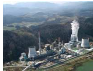
Šoštanj thermal power plant (100% HSE owned)
