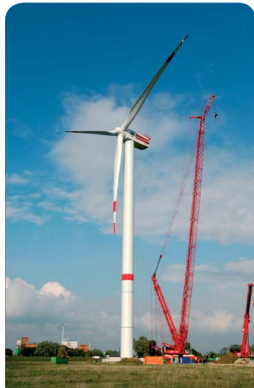
Prototype of RePower 5 MW wind turbine installed at Brunsbüttel, Germany. With a rotor diameter of 126 m, it is the largest wind turbine ever built.
