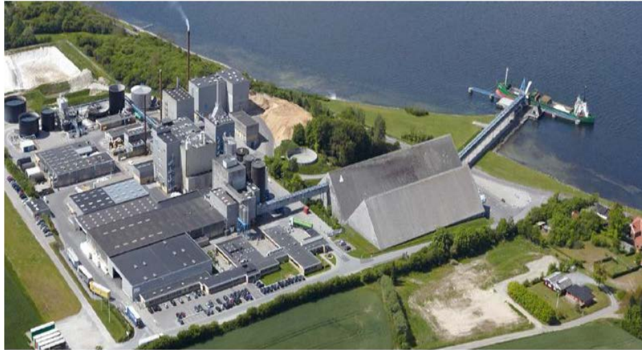
Figure 15 Akzo Nobel salt plant in Mariager, Denmark. The plant has integral biomass steam generation
