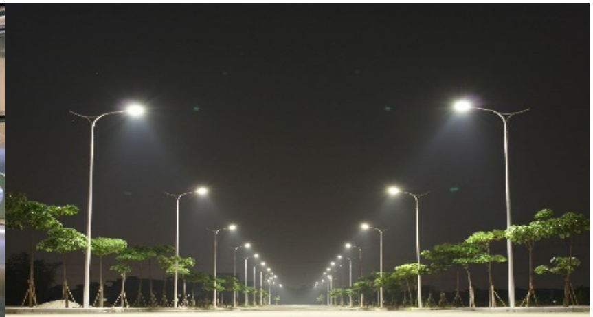
Street lighting upgrades
