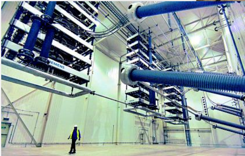
Siemens: Thyristors for HVDC transmission – undersea cable Tasmania – Australia
