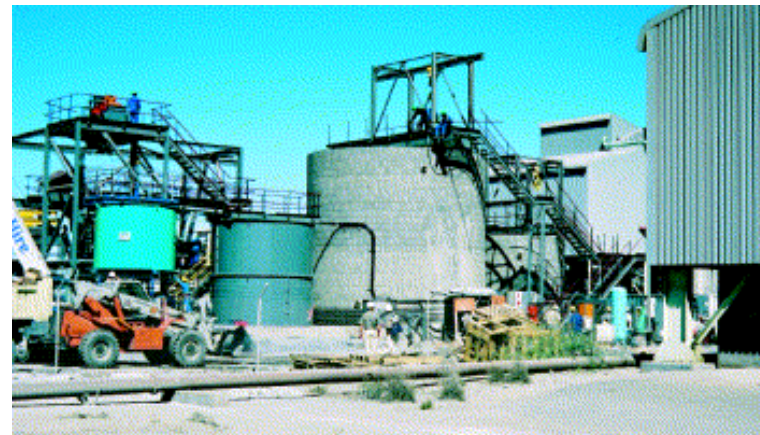
Composite ceramic tanks for thermophile bacteria 300 m 3 Perring, South Africa gold extraction from (arseno)pyrite
