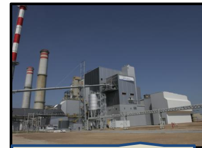
biomass unit in Konin Power Plant
