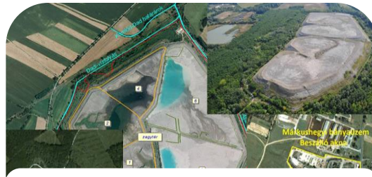
ASH DISPOSAL AREA: UNDER REMEDIATION
