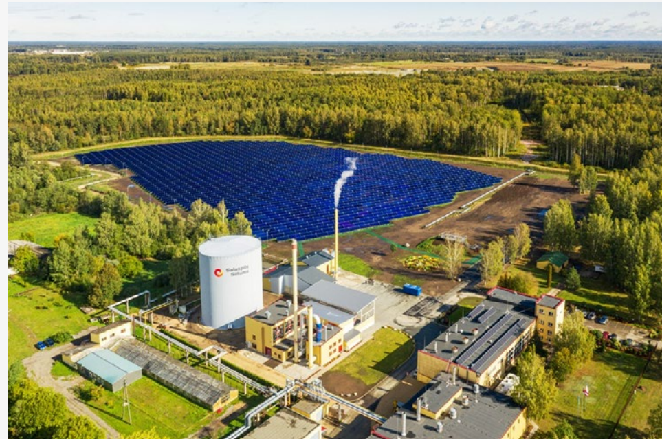
THE SOLAR COLLECTOR FIELD FOR THE DISTRICT HEATING SYSTEM IN SALAPILS, LATVIA
