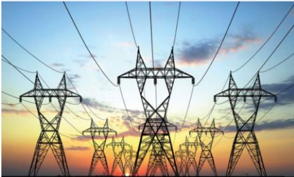
Smart Electricity and Gas Networks
