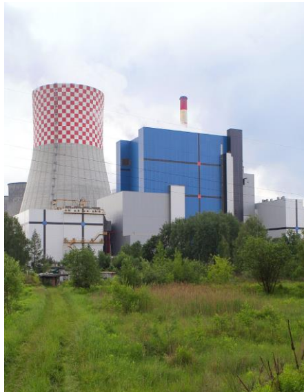
The Lagisza Power Plant in Poland features a 460 MWe Amec Foster Wheeler supercritical, vertical-tube CFB boiler.
