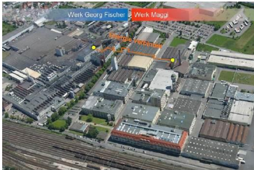
Figure 1.5. Thermal oil pipeline between Georg Fischer Automobilguss GmbH and Maggi
