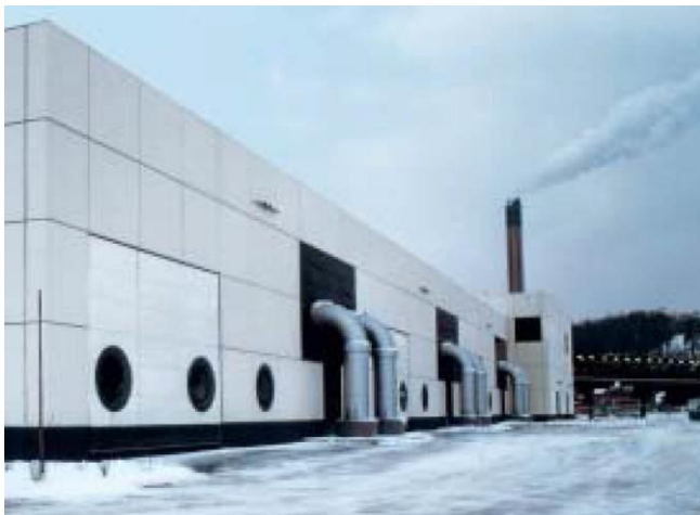
Figure 1.10. Värtan Ropsten pump station building 21
