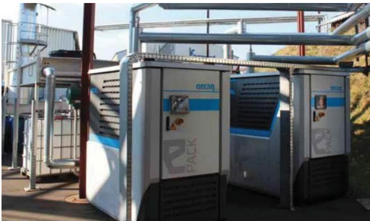
Figure 1.3. Example of an e-Pack ORC unit 9
