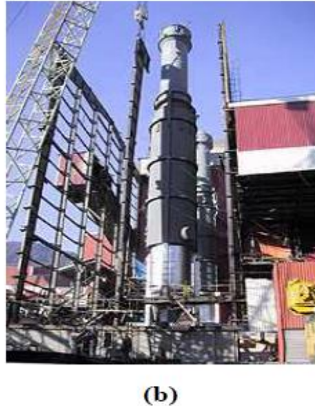
Figure 0.2. (a) Hot medium (e.g. combustion gas) heat exchanger working principle; (b) Heat exchanger mounted on a glass furnace 4
