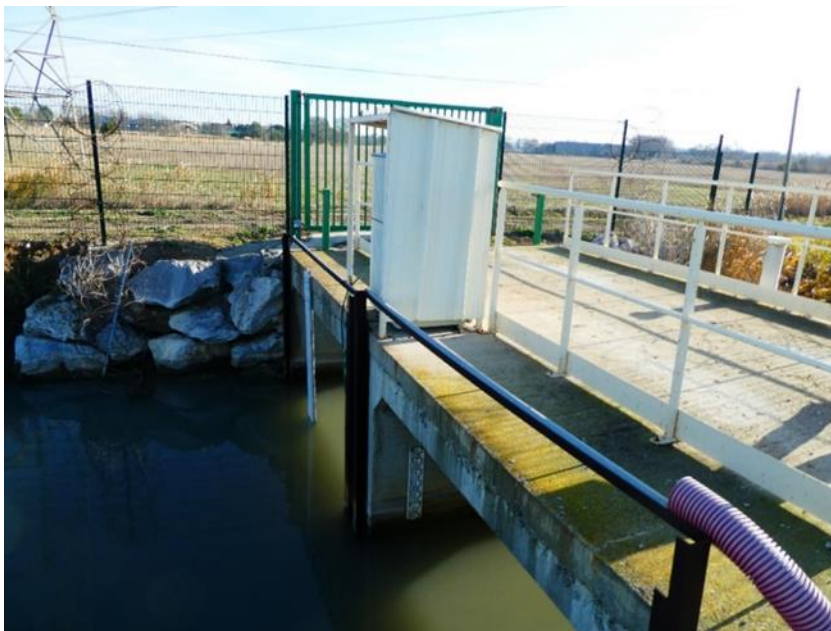
Figure 4. Automatic water sampler
