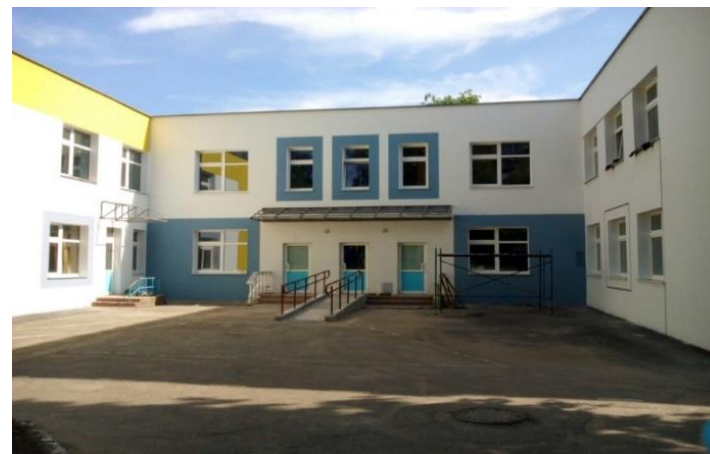
Thermal insulation and double-glazing in kindergarten № 45 in Grodno»
