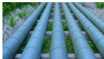
Waste and waste water treatment
