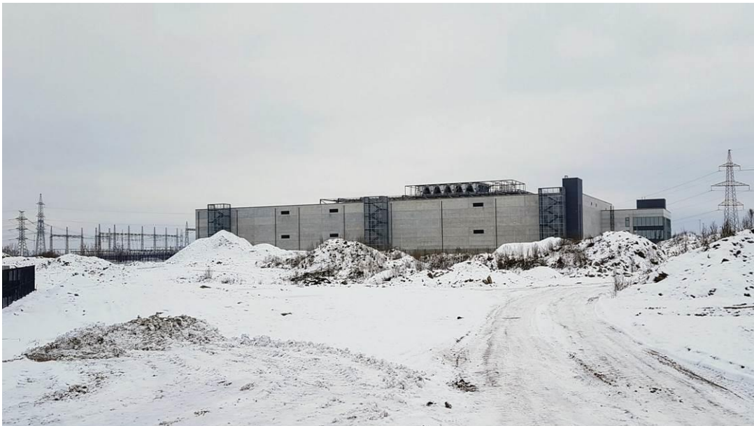
Figure 4.9. MCF Group Estonia Harku data centre next to Harku substation Photo Ü. Kask
