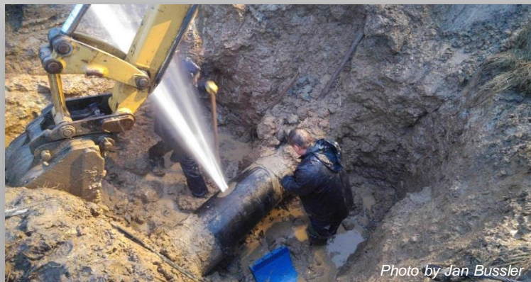
Repair of damage on the Ø 500 mm - public network (March 2017)
