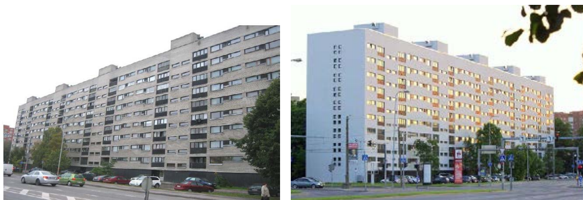
Figure 58: A financed project example- renovation of the apartment block in Tallinn (before and after)
