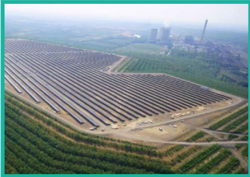
PV power plant in Visonta, HU: 16 MW, 72 500 PV panels
