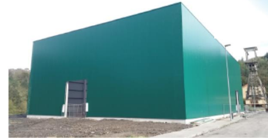
Biomass Logistic Centre in Lieres (under construction)
