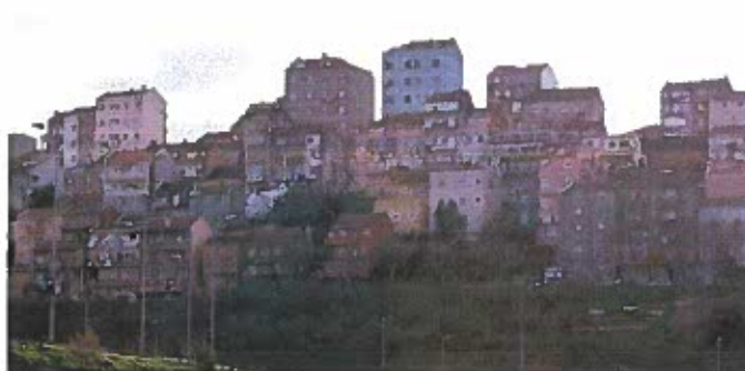
Figure 24 - A view of buildings at Brandoa.
