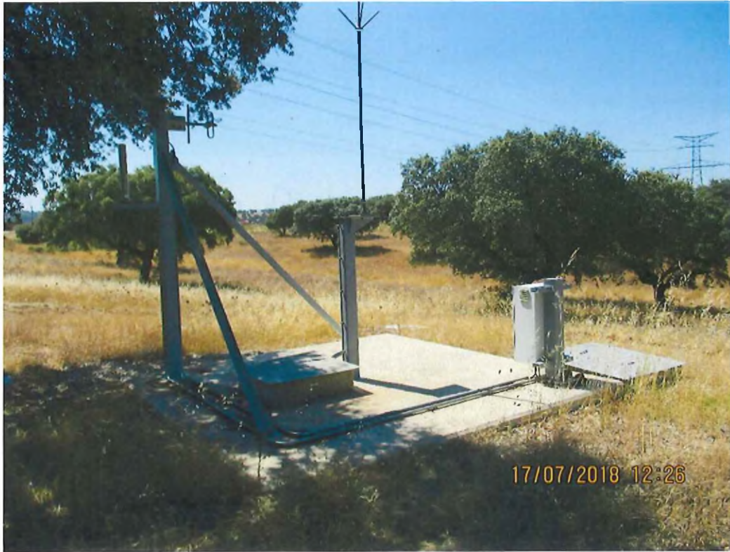
Figure 2: Emergency dose rate monitor
