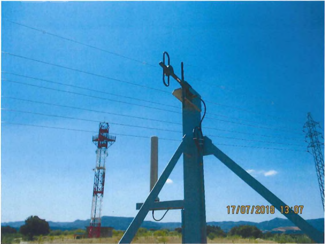
Figure 6: Emergency dose rate monitor
