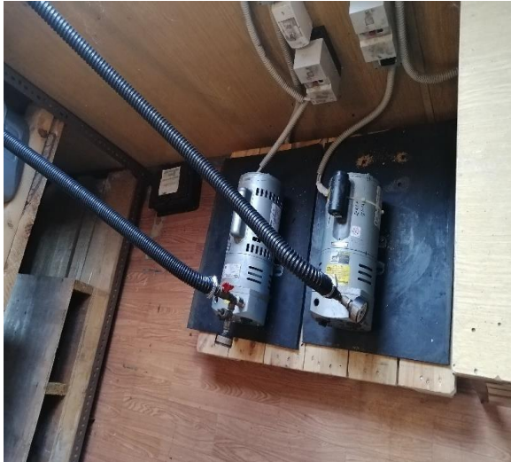
Figure 15. IMROH medium-volume air sampling pumps
