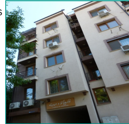
Multi-family residential buildings
