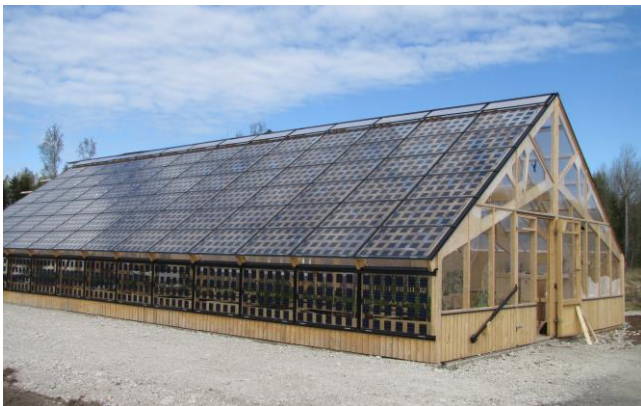
Customized greenhouse, 23 kW, Sweden
